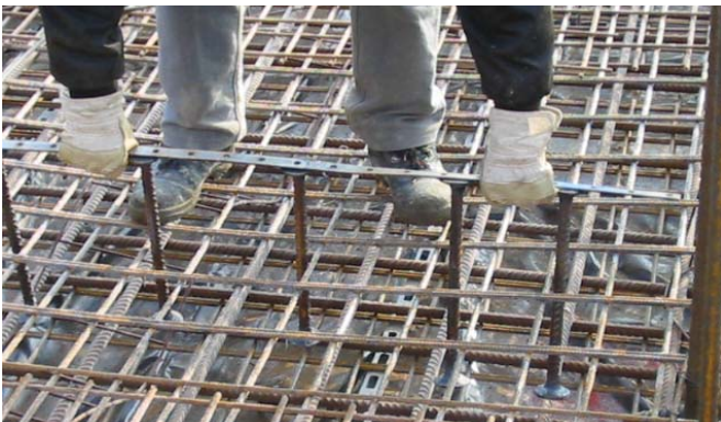
Installation from above for in situ concrete
