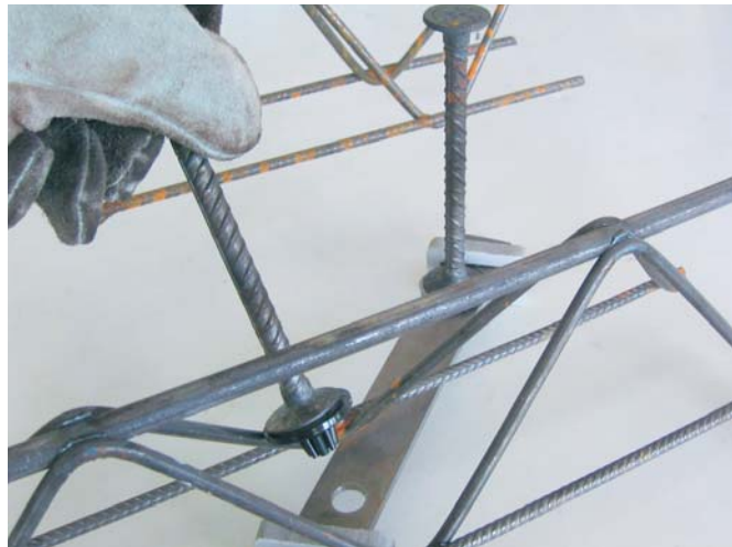
Installation of JDA-FT-KL (the click version)
