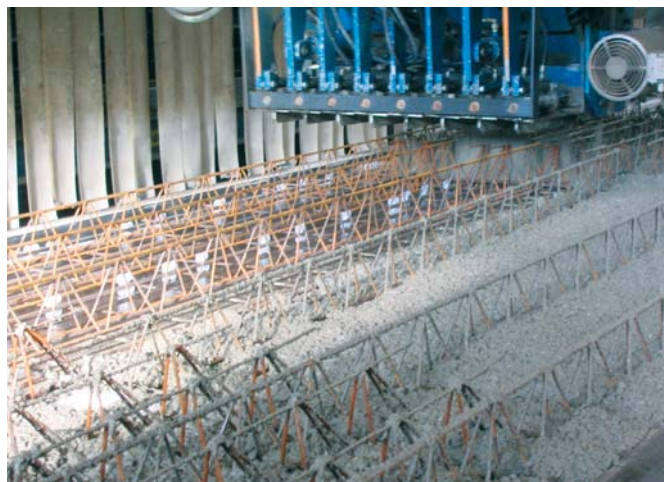
Installation underneath lattice girders in precast elements
